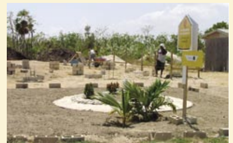
Houses demolished in East End to make way for rebuilding. (top) Foundation laid for one East End house that is undergoing rebuilding. (bottom)
